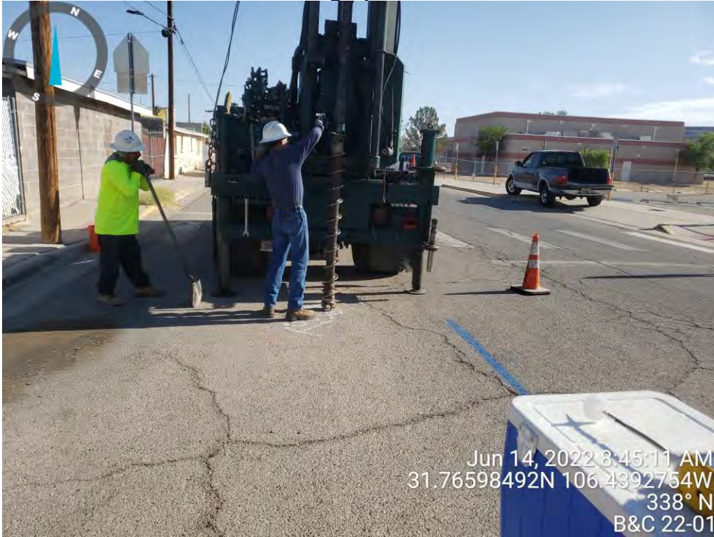
View of initiation of boring operations at B-1.
