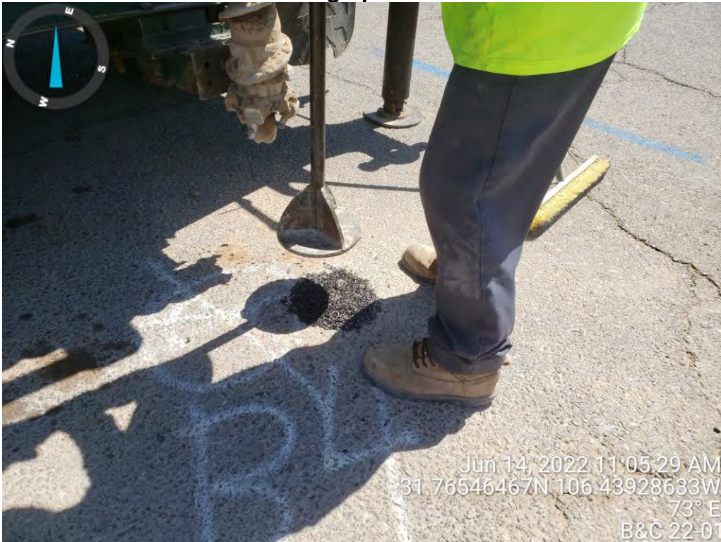
View of boring location being covered after boring activities.
