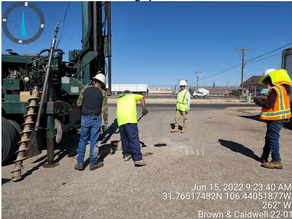
View of B-11 location of auger refusal at Shelter Place.
